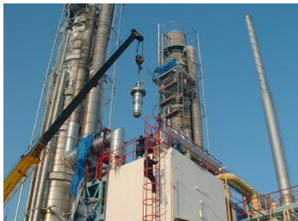
Figure 4. Expander Installation
