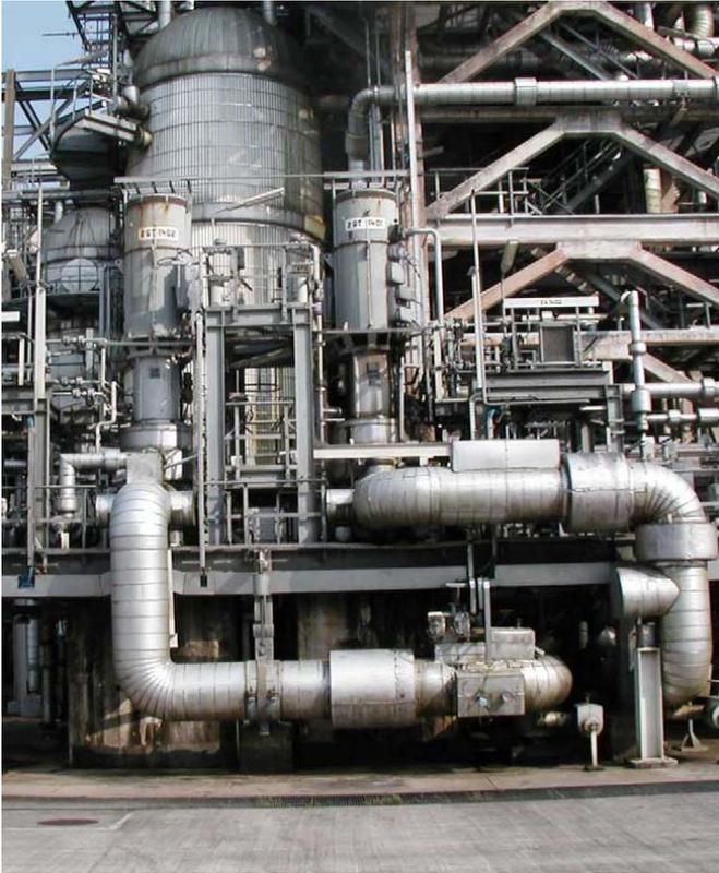
Figure 4: LNG and MR Expanders at an LNG Plant in Nigeria
