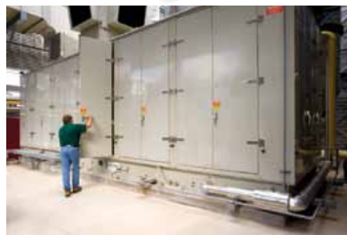
Mercury 50 Generator Set Cogeneration and Distributed Energy Austin, Texas
