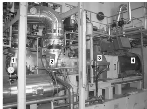
Figure 8: Screw-type steam engine of the biomass CHP plant in Hartberg (net nominal electric capacity: 710 kW el )
