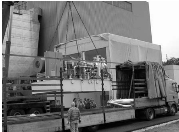
Figure 5: Unloading of the screw-type engine module
