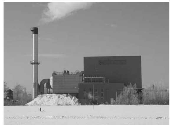
Figure 4: View of the biomass CHP plant in Hartberg (Austria)
